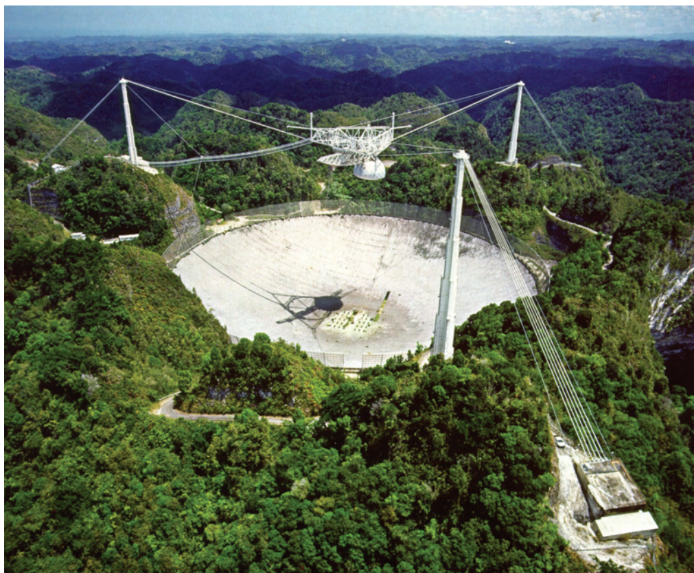
FIGURE 5.10 The 1,000-foot (305-meter) dish at Arecibo, Puerto Rico, is the most sensitive radio telescope in the world. It was used by Projects Phoenix and SERENDIP, and it's currently feeding huge volumes of data to SETI@home. SOURCE: NAIC Arecibo Observatory, a facility of the National Science Foundation.
